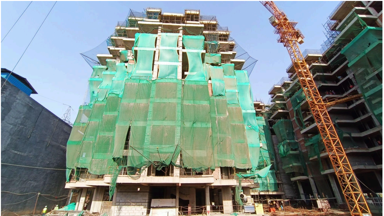
Figure 1. Under Construction Site
